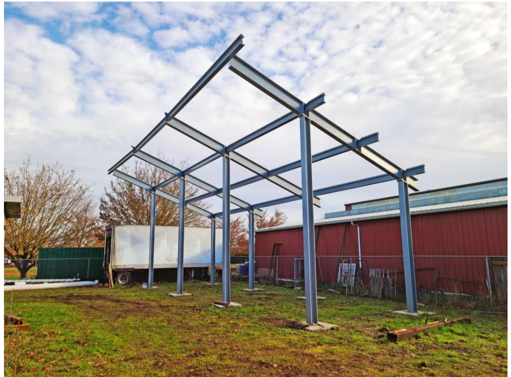
The posts and cross beams for the Linneman Freight Shelter are now in place on their concrete pads. (John Nagy photograph)
