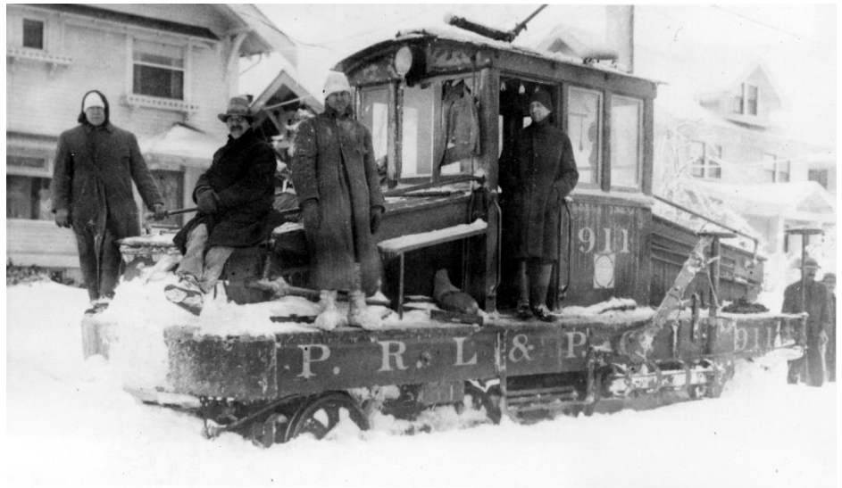
Narrow gauge steeplecab 911 was often equipped with a snow plow during the winter season as seen here on February 13, 1916, on NE Glisan Street in Laurelhurst. She was assigned to the Line & Power Dept during the rest of the year so probably worked as a power station delivery vehicle like single cab flats 915 and 916. No. 911 was built in 1906 and retired in 1946.
