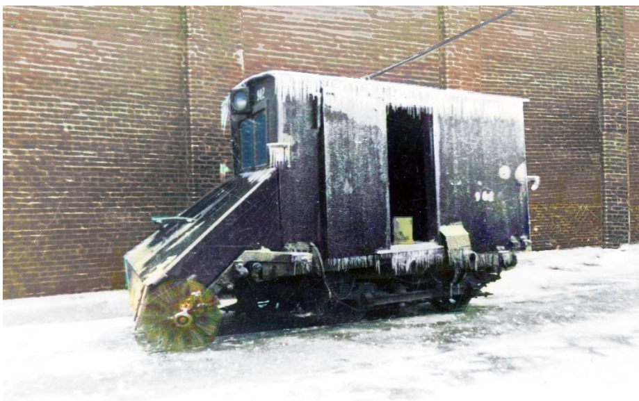
Snow sweeper No. 902, seen here at the Piedmont Car barn in the 1940s, was one of four narrow gauge “brooms” built by the City & Suburban Railway during 1900-1901. They were equipped with two GE-58 motors for propulsion and two Sprague motors for the broom. No. 900 was retired in 1916 but the other three lasted until 1946. (Charles Hayden photograph)
