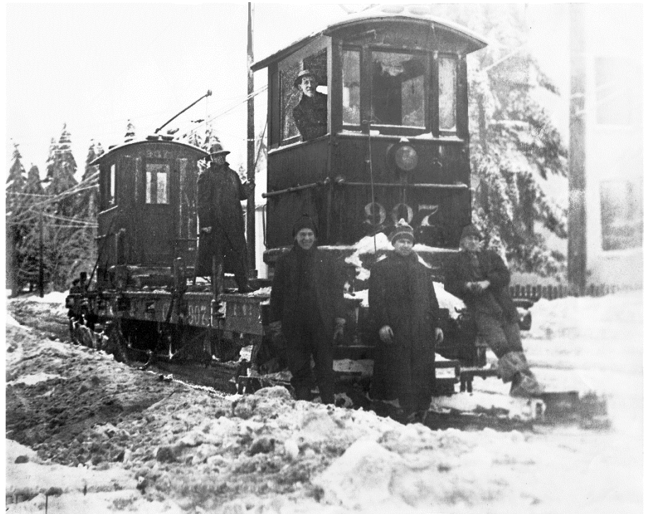
What PRL&P designated as Class X "construction motors" were outfitted with plows during the winter and, along with the sweepers, did the lion's share of snow removal. No. 907 was a two-cab flat built by PRL&P in 1913 and rebuilt in 1931. She lasted in service until 1948. Note the weather-proofed boot covers on some members of this happy team.
