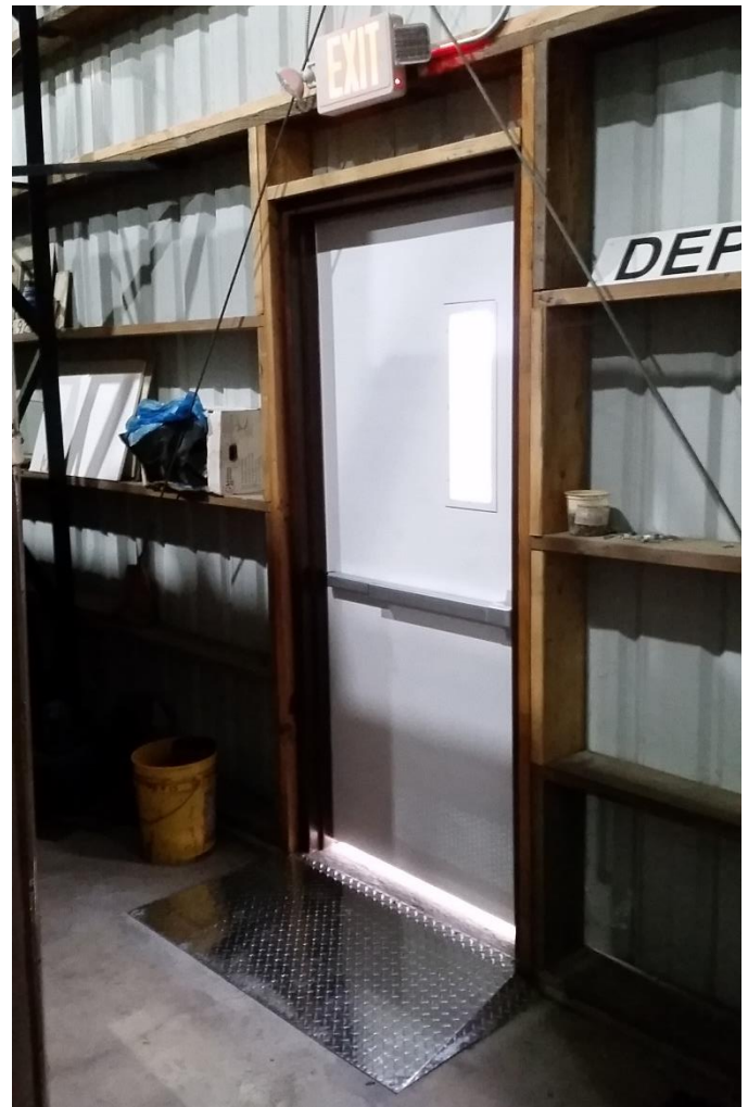
New emergency exit with diamond plate and concrete ramp.
