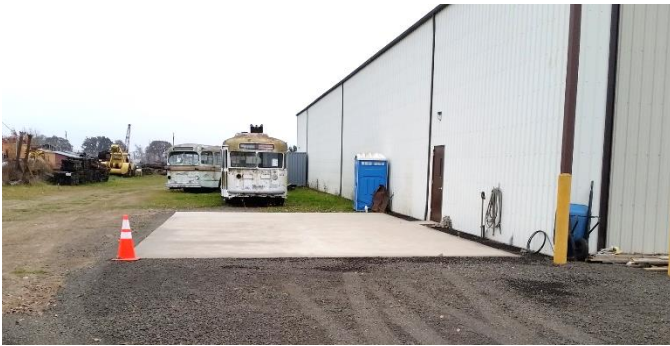
New concrete parking lot with reserved handicapped parking.
