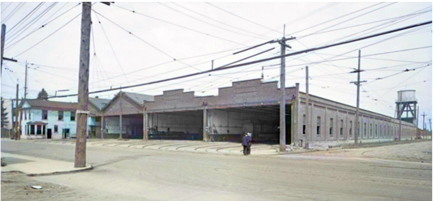
It must be rush hour because two carmen are conferring in front of empty bays A, B, C, and D in this undated picture taken at the Piedmont Car barn on the corner of N. Killingsworth Street and N. Mississippi Avenue
