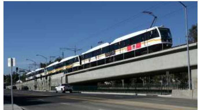
Los Angeles Metro. On tracks once travelled by Pacific Electric and Southern Pacific on the right-of-way of the old Santa Monica Airline, an LA bound set of Siemens P2000 LRV light rail cars climbs towards to grade separated La Cienega station.
