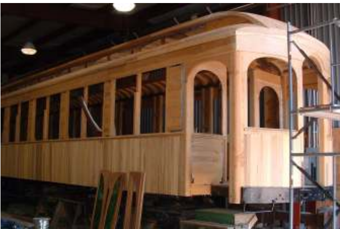
A car similar to car 65 being restored. This is typical of the reconstruction process at the Black Hills Central shops
