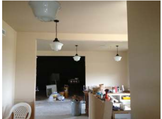
Sheetrock and painting complete, new light fixtures installed.
