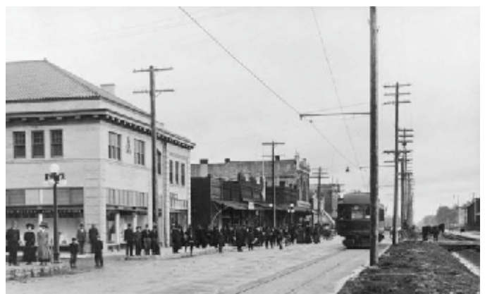
Oregon Electric train at end of the track at the corner of Arthur Street looking North on Front Street in Woodburn, Oregon. The Southern Pacific Railroad is on the right. The light beige building on the left is still standing today. This picture was taken on opening day in 1912.
