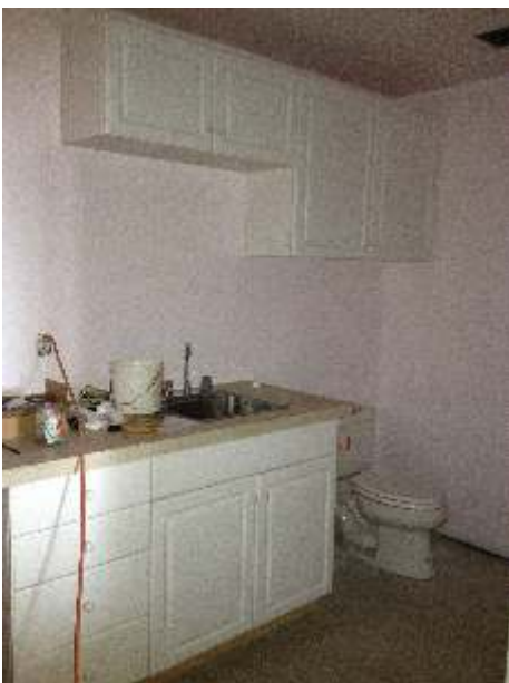
New cabinets , counter top, and stainless steel sink in the restroom.
