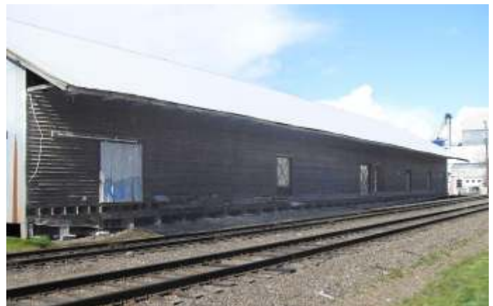
Donald freight house on 3/26/2011. This former OE freight warehouse at Donald is typical of the warehouses in the various communities in the Willamette Valley. The warehouse is currently being used by local farmers, not the railroad.
