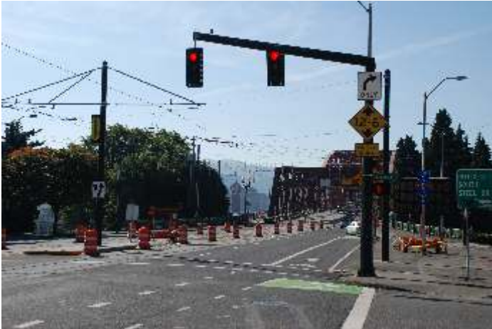
East approach to Broadway Bridge--tracks and overhead in place
