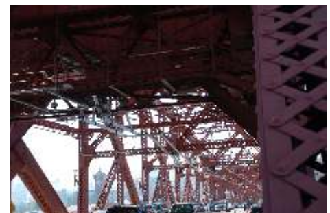
Overhead almost complete. Union Station can be seen in the background
