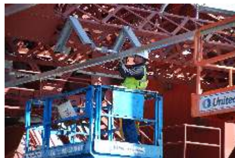
Attaching insulators and overhead support structure
