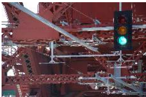
Detail of overhead attached to bridge structure.
