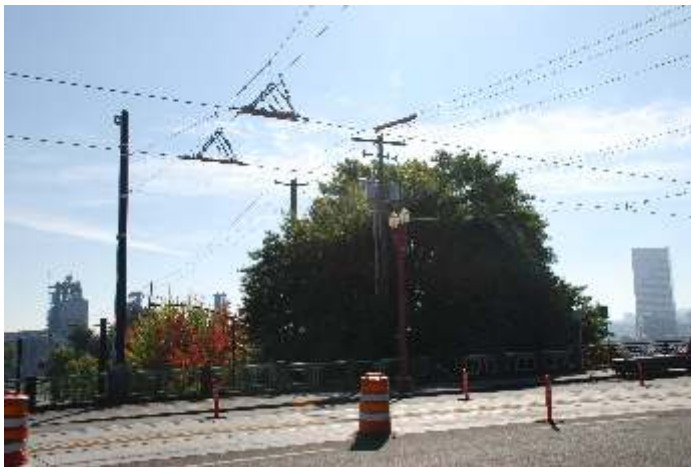
East ramp up to Broadway Bridge showing overhead transition.
