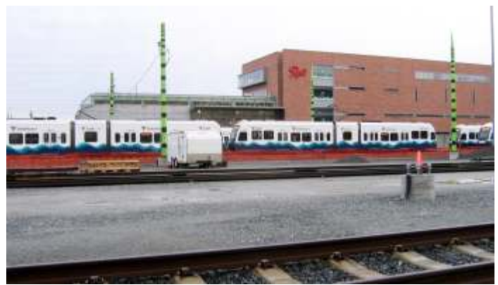
Looking at the Eastside of the Sound Transit Light Rail maintenance shop and rail yard. In the foreground is where Sound Transit is expanding their rail yard.
