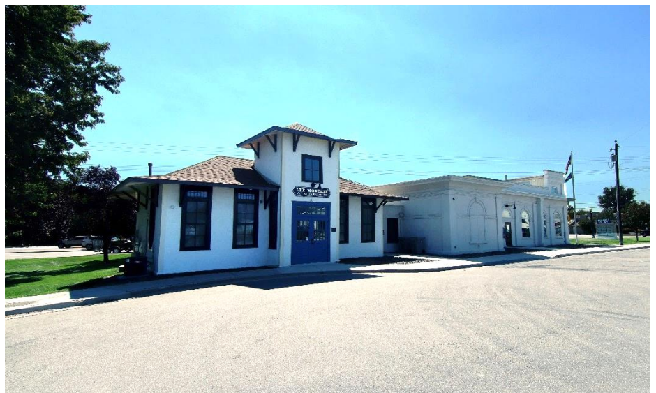
Middleton station, with the former substation next to it, is today home to the Lee Moberly Museum and Event Center. Lee Moberly was the Middleton postmaster and a local historian. (Mark Kavanagh photograph)
