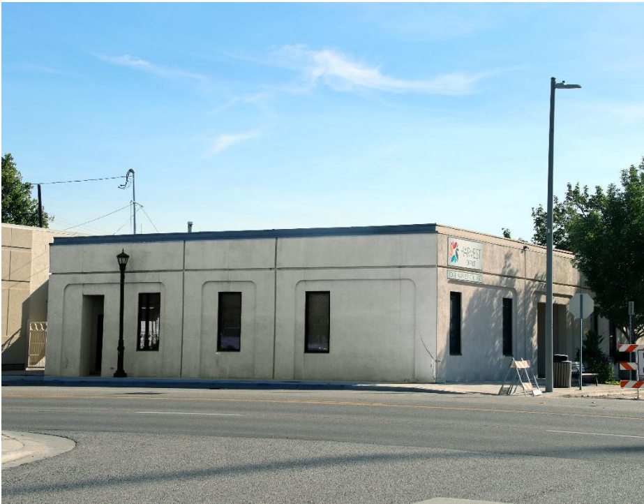
Meridian station at the corner of N. Meridian Road and East Idaho Avenue now serves as college classrooms. (Mark Kavanagh photograph).
