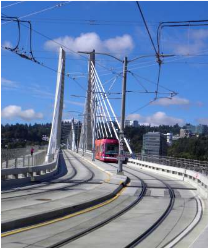
A-Loop streetcar headed west across the Tilikum Crossing
