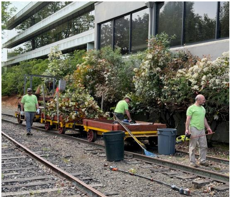
Chris Cox, Jay Weitman, and Ethan Perkins clear brush from the WST Carolina Street siding (Gage Geist photograph).
