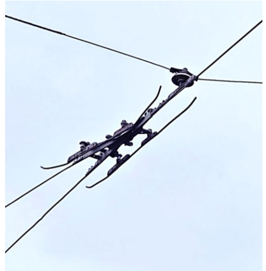
Closeup of the yard switch frog showing the addition of pantograph-capable bars. (Mark Kavanagh photograph)
