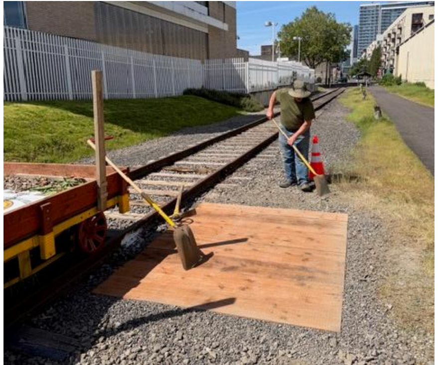
Bob Davidson installing the new temporary platform at what is known as the "Tesla Crossing" due to the nearby service center. (Gage Geist photograph)
