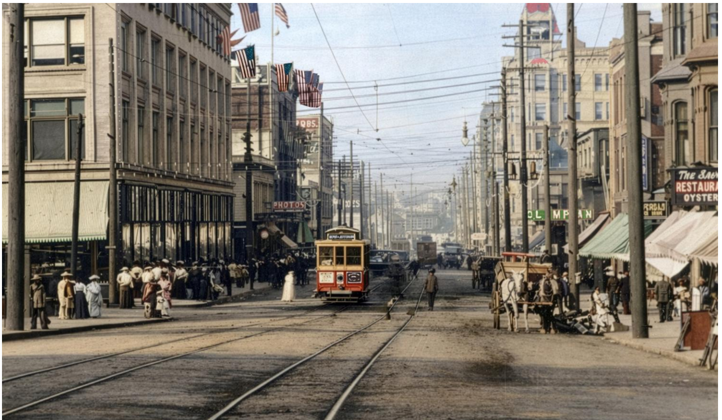
An electrified Portland Heights line cable car is seen southbound on Fifth Avenue at the intersection with Morrison Street during the late 1890s. The Meier & Frank department store is at left and on the right are the Savoy Restaurant, the Olympian tavern, and the Perkins Hotel. The Perkins Hotel was built by a cattle baron and featured a gilded cedar steer on its roof. Note the absence of automobiles.
