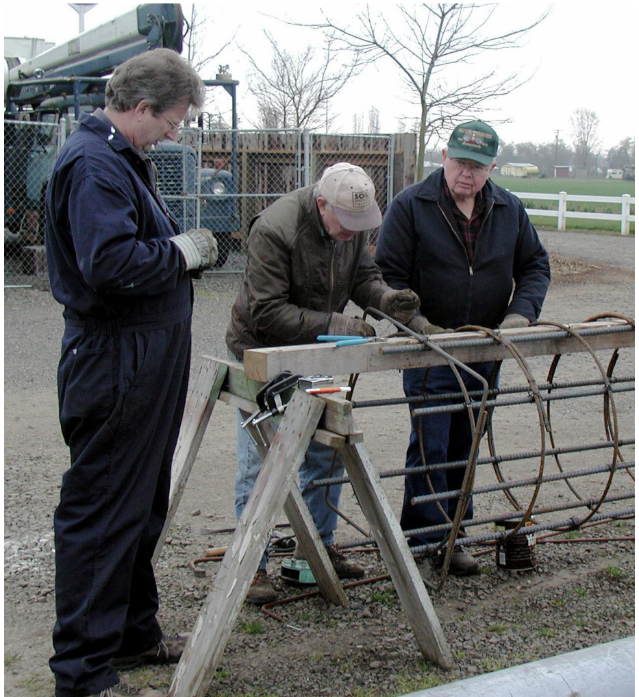
Peter Kloosterman, Bill Binns, and Bob Terkelsen building rebar forms for the overhead poles.
