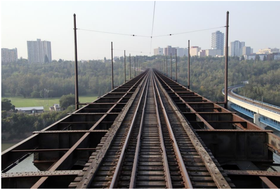
A view of the tracks on the High-Level Bridge. How would you like to do track or overhead work here? (Mark Kavanagh photograph)
