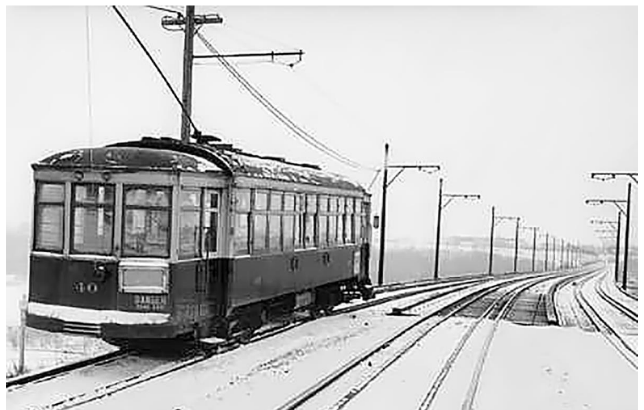
Edmonton Radial Railway No. 40 is using the left-hand track as it heads northbound across the high-level bridge in 1920. (Wikipedia)
