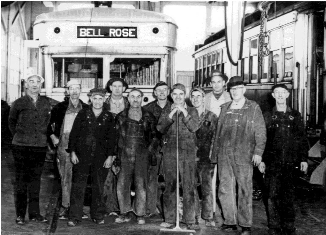
The entire Portland Rail & Terminal Division maintenance crew is seen inside the East Portland Yard shop. Master Mechanic Roy E Reinke is at far left and Jefferson Christie at far right. The two streetcars behind them include one of the three "Yaks" and one of the 1092-1102 series wooden cars.
