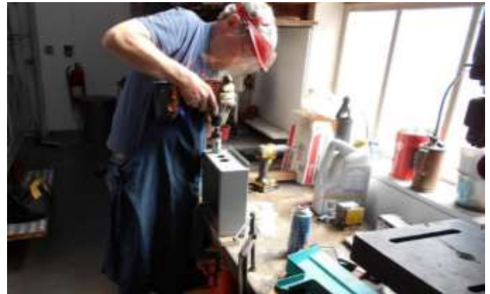
Dave Rowe drilling conduit fitting holes into one of the inverter motor disconnect boxes.
