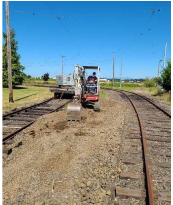
Evan Burroughs removing gravel between the mainline and yard curve so that the curve can be realigned. (John Nagy photograph)
