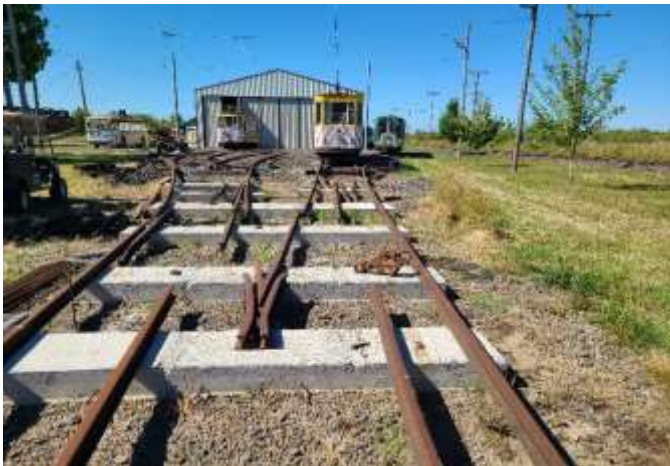
Volunteer Crews have started to reassemble the yard tracks in front of the carbarn. (John Nagy photograph)
