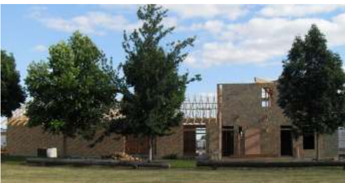
Walls taking shape on July 2nd.
