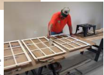
John Nagy painting mullions for the first floor windows.
