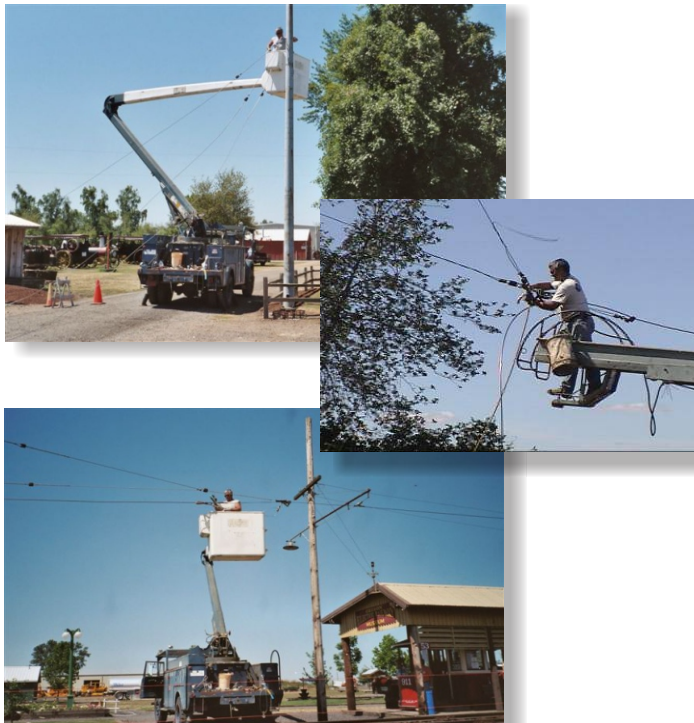
Greg working in the lift bucket on overhead for the extension to the Brooks museum depot. Another photo shows him attaching pull off wires for curve between sawmill and truck museum. The work on the rail extension was in 2003.
