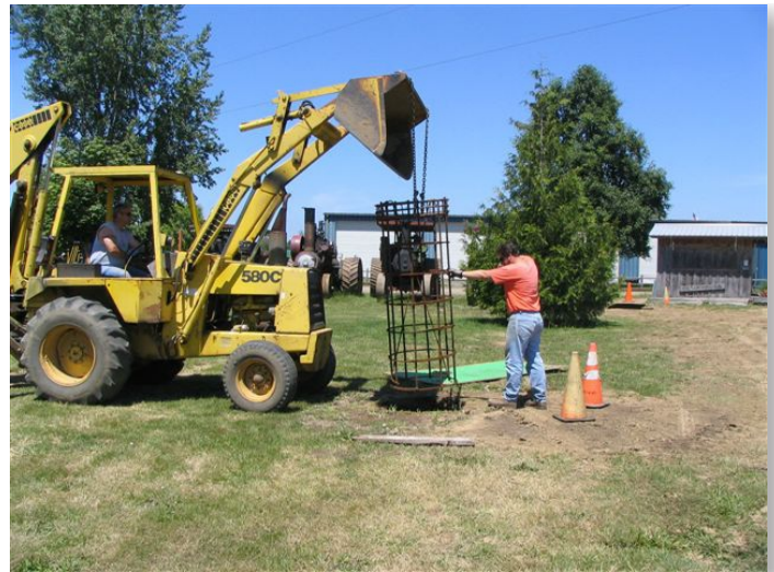
John Nagy is working with Greg placing rebar cage for the foundation for the steel poles.
