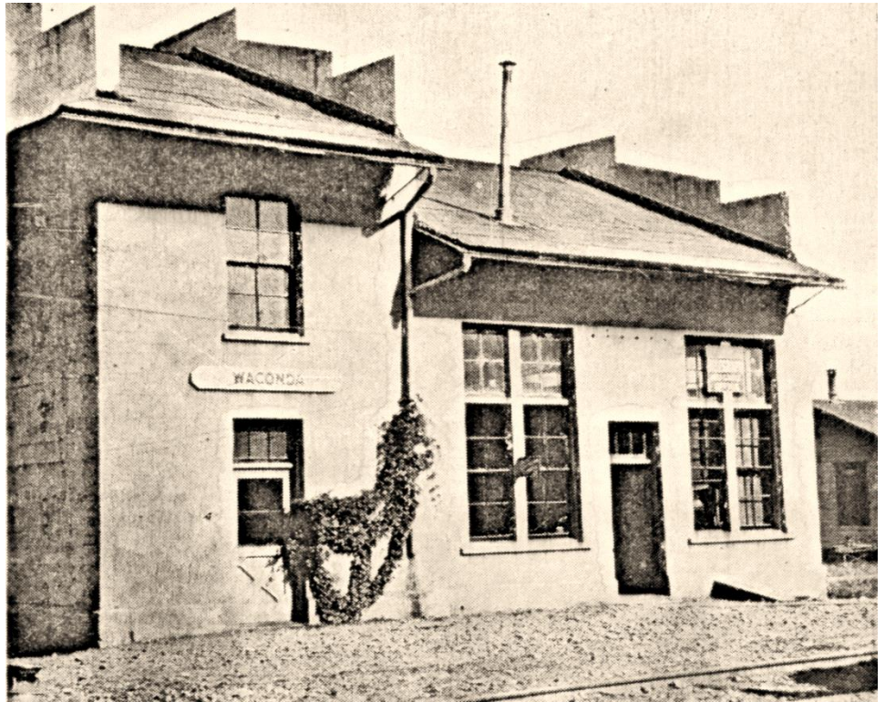
The Oregon Electric Railway's Waconda station was another that featured a combined substation and agent's office. (illustration from 1915 Electric Railway Journal).
