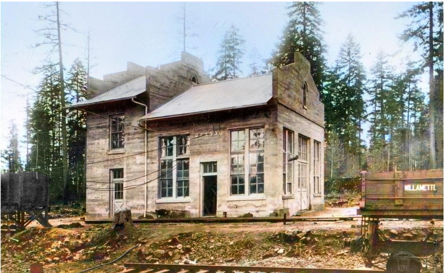
Wacanda, seen here during construction, was a combined substation and station agent's office. Located 11 miles north of Salem, the station had a two-story-high voltage compartment, electrical room, and a one story ticket office with waiting room.
