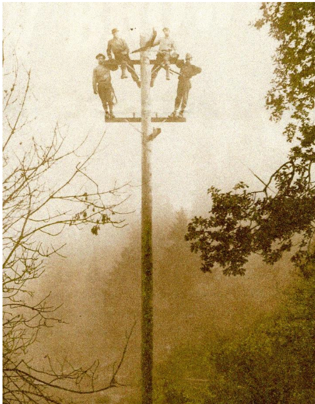
In this view of Charles Chaney and fellow line workers high atop a pole it is easy to see why the job of lineman was considered one of most dangerous professions. Between 1890 and 1930 one in three linemen were killed on the job. (Janice Becker)
