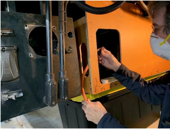
At the corner of the battery will be access to the main fuse and disconnect switch. The disconnect switch will have linkage rods to each side of trolley to be used by first responders if ever needed. Bob Simpson is pictured with a COVID-19 mask.
