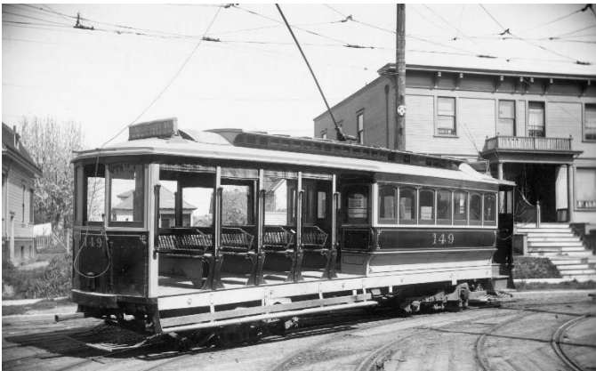
No. 149 (originally 78) was an 1899 product of the Hand Manufacturing Company; whose factory was the first to build streetcars on the West Coast. The "California" style half-open body was created by splicing together two horsecars. It is seen at the Ankeny Car barn during the Portland Consolidated Railway years (1904-05).
