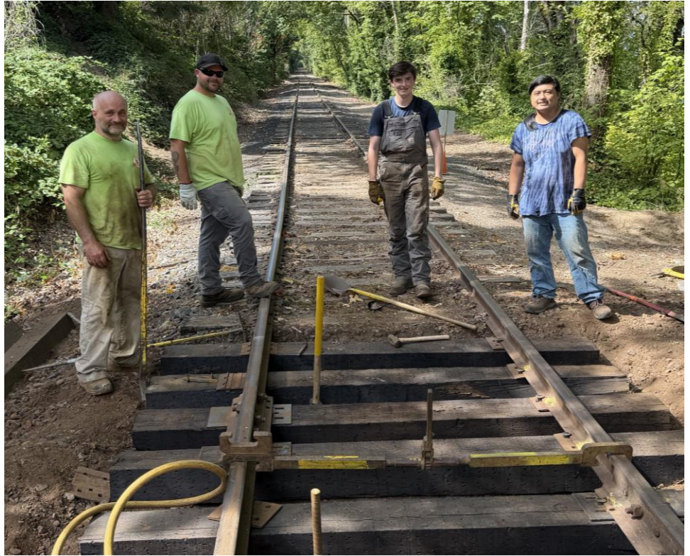
The Willamette Shore Trolley track crew are preparing to spike the last ties in Powers Marine Park. Left to right: Ethan Perkins, Chris Cox, Jack Higgins, and Theodora Wong. Driving the final “golden spike” can be seen at lower left. (Gage Geist photograph)
