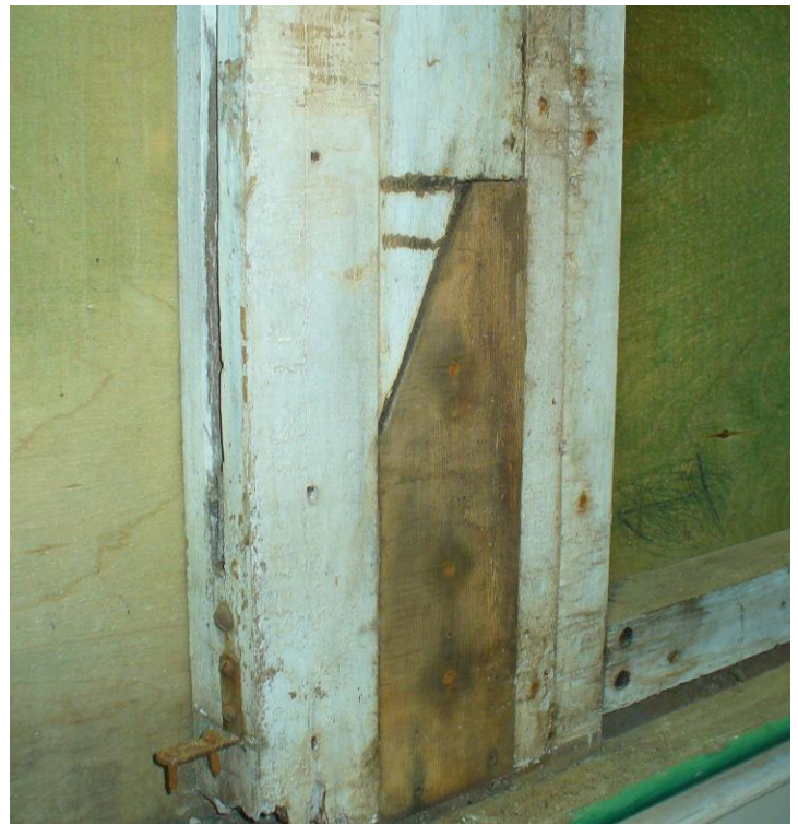
The support column on No. 48 after it had been repaired by Gene Fabryka. (Pete Manuelle photograph)
