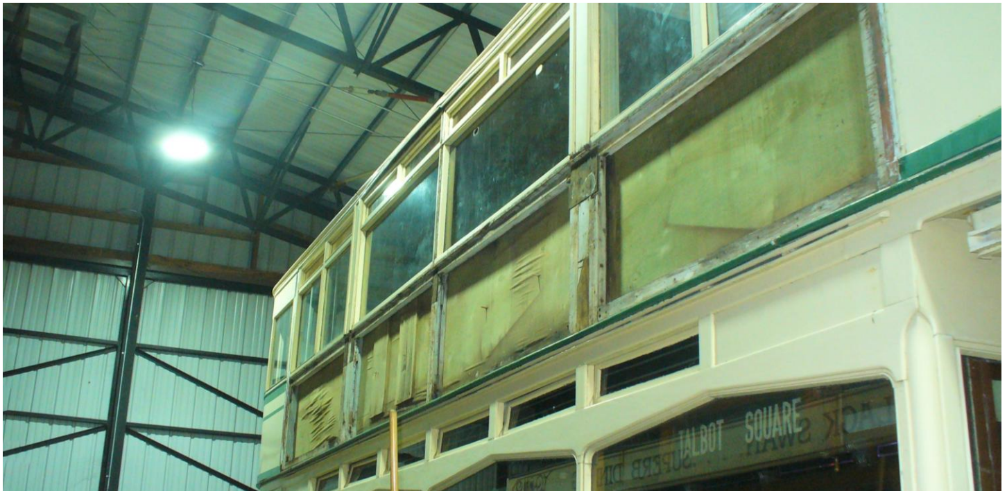
The outer panels on No. 48 were removed from the upstairs wall for evaluation and repair. (Pete Manuele photograph)
