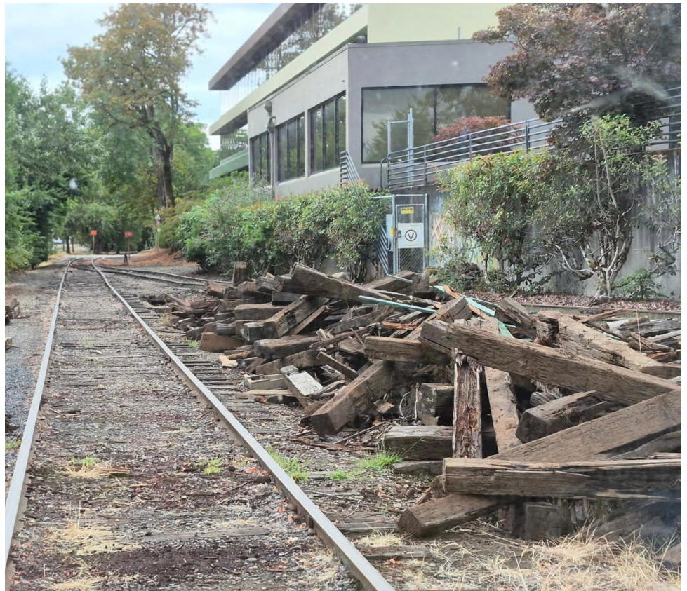
The massive pile of old ties removed from Powers Marine Park at the Carolina Street Yard. (Gage Geist photograph)
