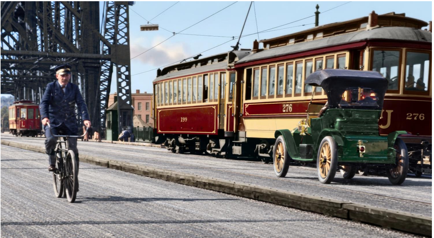
Three modes of transportation are displayed in this photograph taken on the new Steel Bridge in 1912. At right, a Pierce-Arrow runabout is about to pass a two-car St. Johns line train consisting of interurban motor 199 and trailer 276. A bicycle messenger is approaching the camera on the left, while a Lower Albina line trolley can be seen in the distance. (from Portland Memories on Facebook, colorized by the author)
