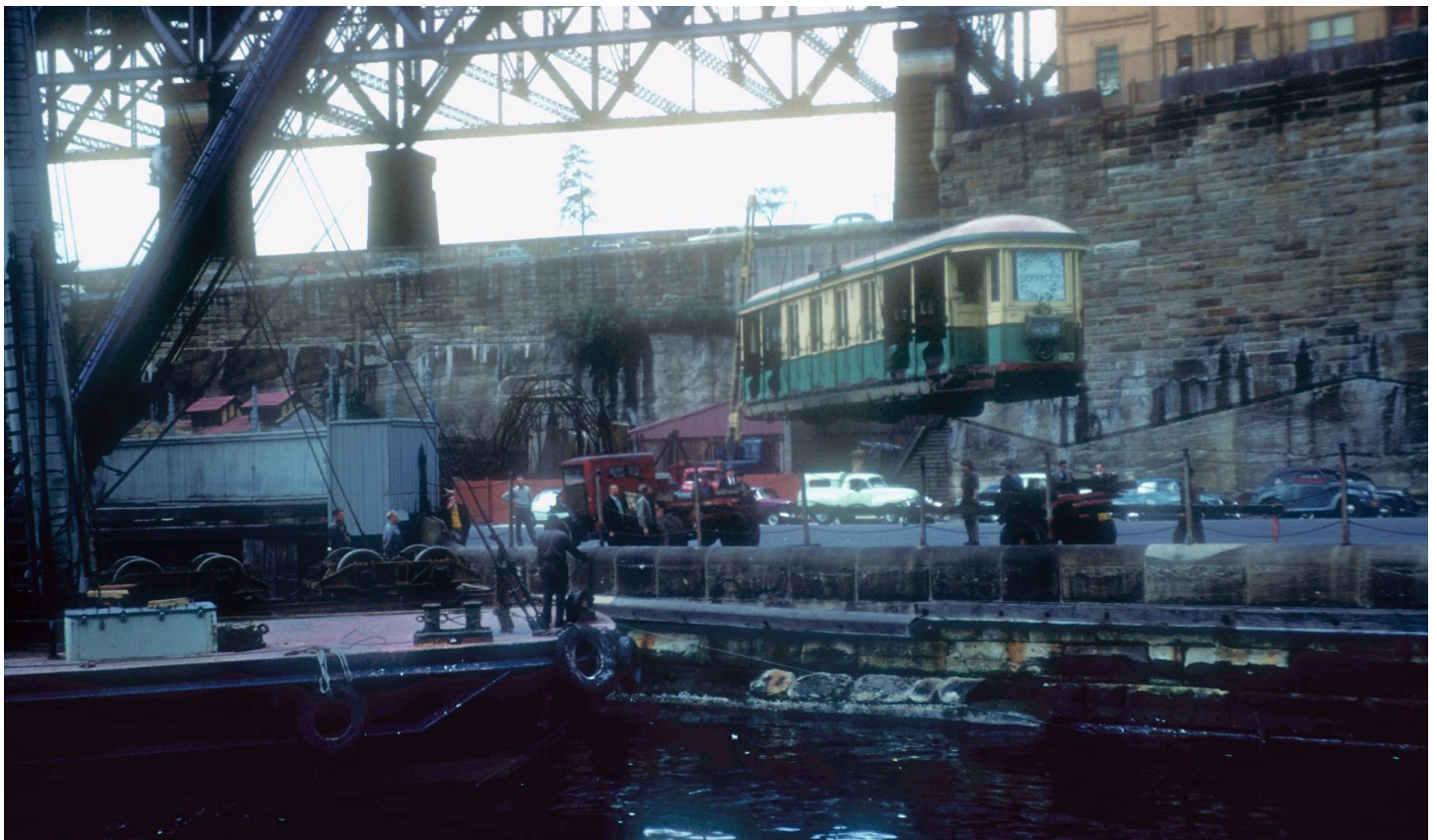
The body of car 1187 is lifted onto the steamer Ventura on July 16, 1959, while the "bogies" (trucks) wait on the crane barge at left. The Sydney Harbor Bridge looms in the background.
