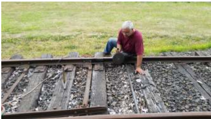
Greg Bonn repairing switch point
