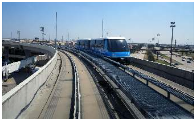
Skylink at DFW Airport
