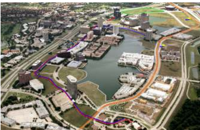
Las Colinas Area Personal Transit System (APT) system map (red and blue) with DART route shown in orange.
