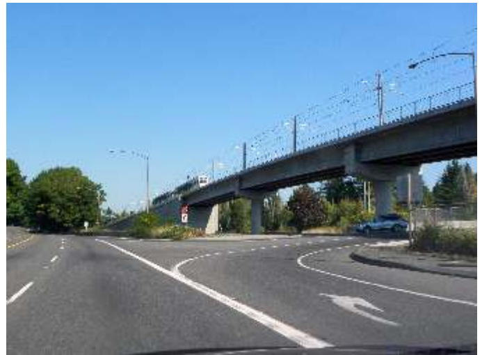
One of the many elevated flyovers on the Orange Line to Milwaukie. This one is located at S.E. Tacoma St in Milwaukie. Tacoma runs from McLoughlin Blvd in Milwaukie to I-205 in East county.
