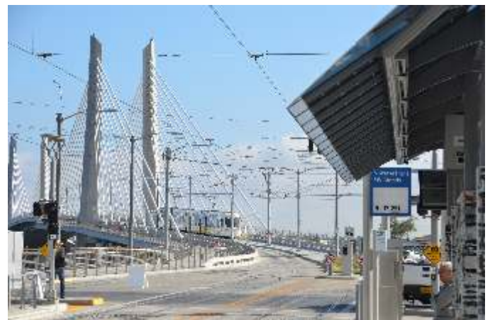
MAX Orange Line from Milwaukie leaving Tilikum Crossing about to stop at S. Waterfront/SW Moody station.
