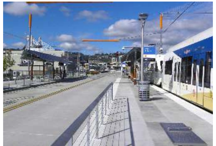
OMSI-SE Water station at the eastern side of Tilikum Crossing. Type 2 LRV headed south to Milwaukie and Type 4 headed across the Tilikum Crossing to downtown Portland.
