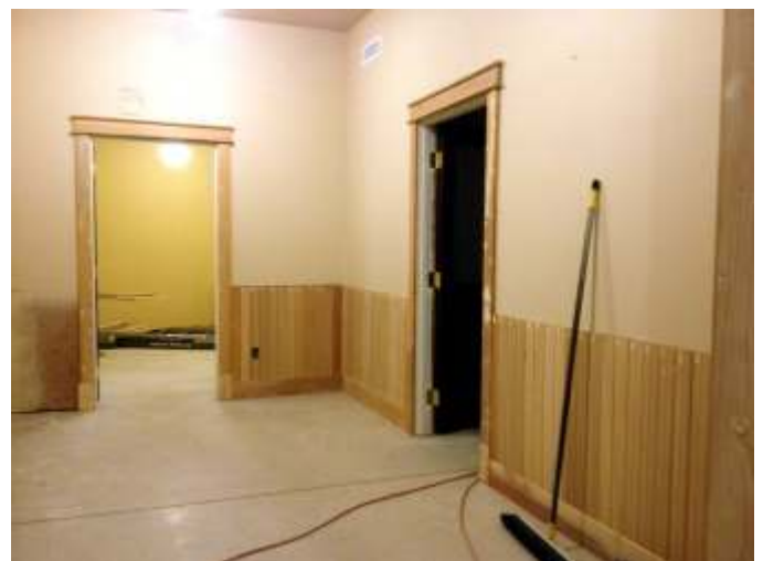
Looking toward library from entrance hall.
