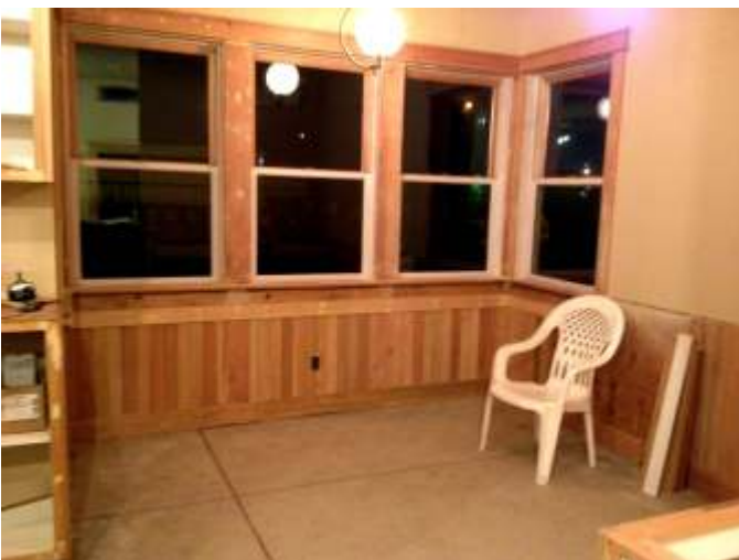
Bay windows, dispatcher's desk area.
