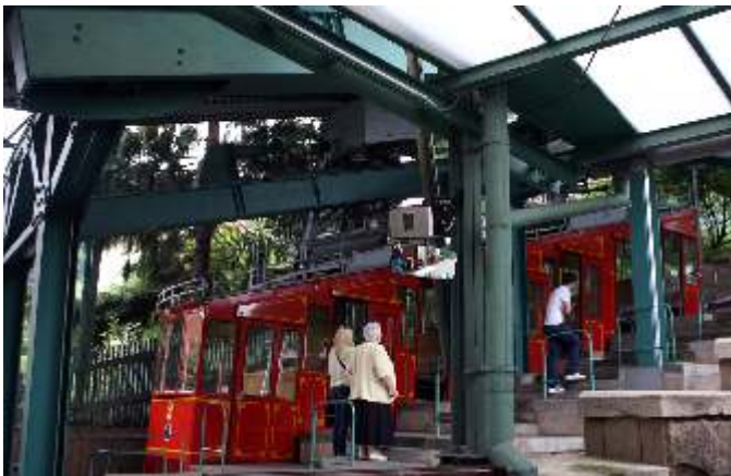
Schebebahn at the lower station
