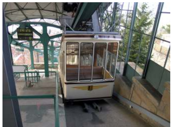
Schebebahn from upper station
