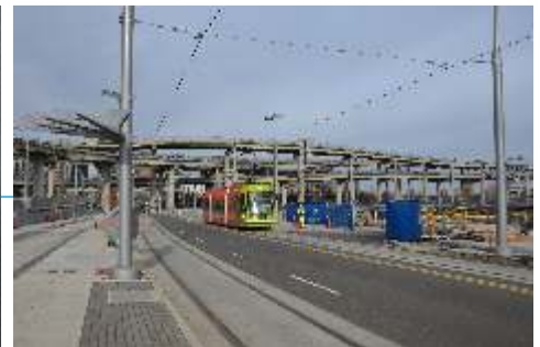
SW Moody Ave. looking north.
