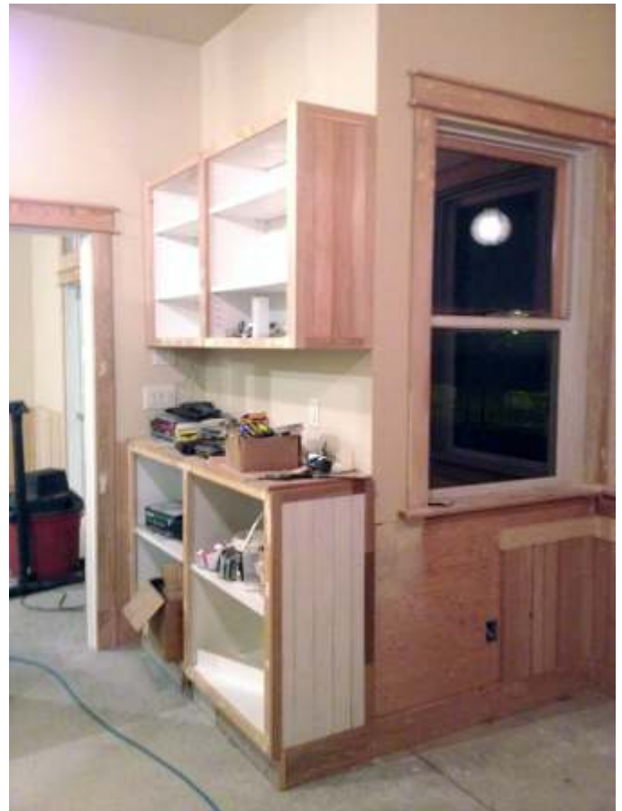
Cabinets behind ticket counter.
