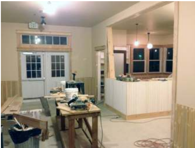
Entrance hall looking toward ticket counter.
