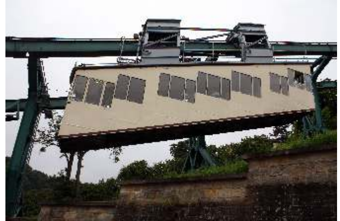
Schebebahn as seen from below
