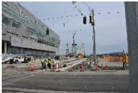
Construction of the west ramp to the transit bridge along SW Moody Ave.
