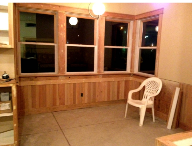
Bay windows, dispatcher's desk area.
