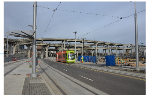
SW Moody Ave. looking north.
