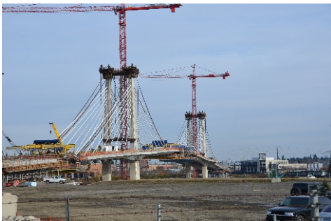
Transit bridge between OMSI on the east side and south waterfront on the west side closing the gap. When completed, this will complete the loop line.
