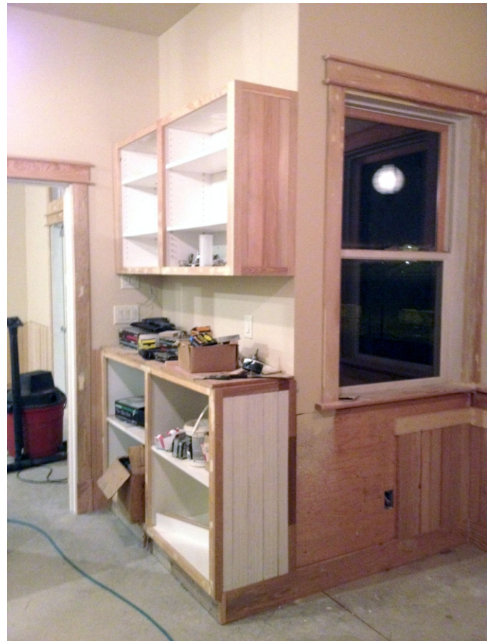
Cabinets behind ticket counter.
