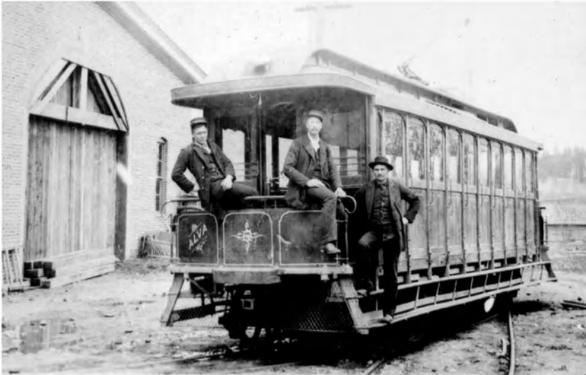
The East Side Railway's first interurban, "Alva," is said to have been named for the Spanish Duke of Alba, who visited the railway while it was being built. It was a Vulcan convertible built locally in 1891. (Al Haij Collection).
