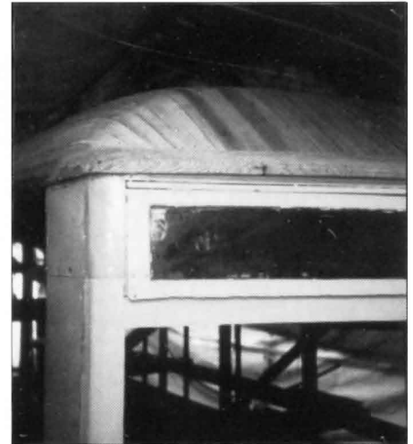
Fresno Birney 74 has received a new roof while undergoing restoration in Edmonds, WA (Tom Mendenhall Photo)
