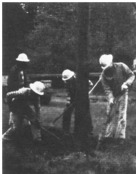
PNB volunteers, and our own Mike Parker, installing new poles on the mainline at the Trolley Park. Left to right: Larry Smith, Don Norman, Mike, and Vic Minkler. (Carolyn Novak photo)
