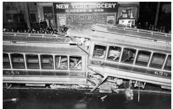
This collision took place in 1915, when empty Sunnyside car No. 649 slipped its brakes during a layover at Southwest 13 th and Hall streets, travelled several blocks downhill to Southwest 11 th and Morrison, where it hit standing Mount Tabor car No. 659. Both trolleys rose in the air on impact and then crashed down on each other, seriously injuring several passengers. (Thompson collection).
