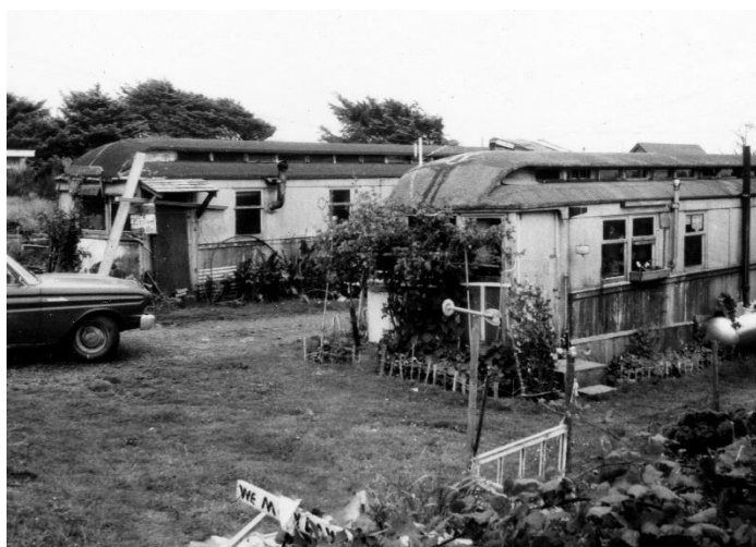
1065 and 1067 as beach cabins at Tolovana Park in 1975. These cars had train doors, which were removed when rebuilt for one man service. (Bill Hayes photograph)
