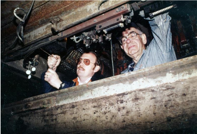
OERHS members Keith Stephenson (left) and Al Nelson install a new voltage regulator on PCC No. 1159 at the Trolley Park on May 9, 1981 (Thompson photograph)
