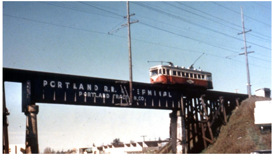
No. 4012, or sister 4014, is crossing the trestle over McLoughlin Blvd. during the 1950s. These two cars were converted from narrow to standard gauge for service on the interurban lines. The former "Broadways" began work on the Oregon City and Bellrose lines in 1950, but 4014 was found to be unsatisfactory and retired by 1954. Car 4012 lasted until the end (1958) and is now a mainstay of the OERHS collection.
