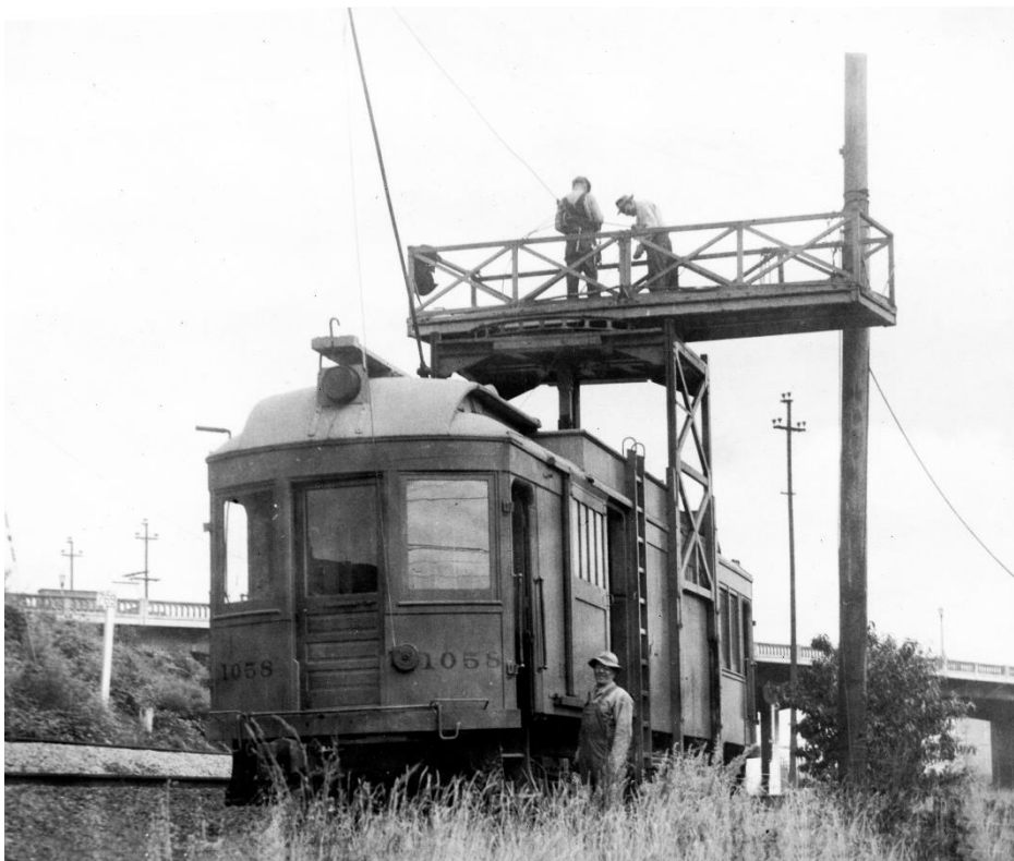
The overhead is down (or perhaps being removed) in this 1950s view of line car 1058 at work. The photograph is attributed to veteran motorman Fred Blaisdell and looks southeast toward the Grand Avenue Viaduct from a point near the East Portland Yards.
